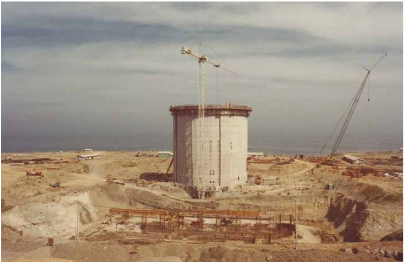
Wolsong I under construction
