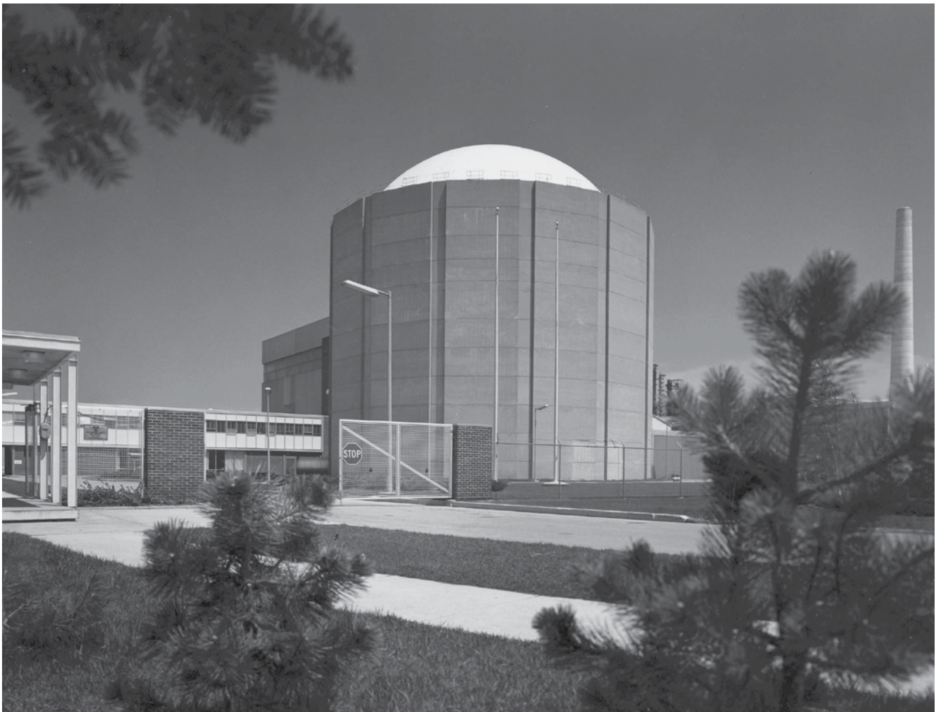
Douglas Point was the full scale prototype of the CANDU reactor system
